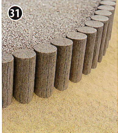
CEDAR POST RETAINING WALL
