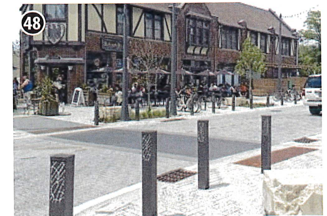
FLUSH DECORATIVE PAVING AREA, CURBLESS
