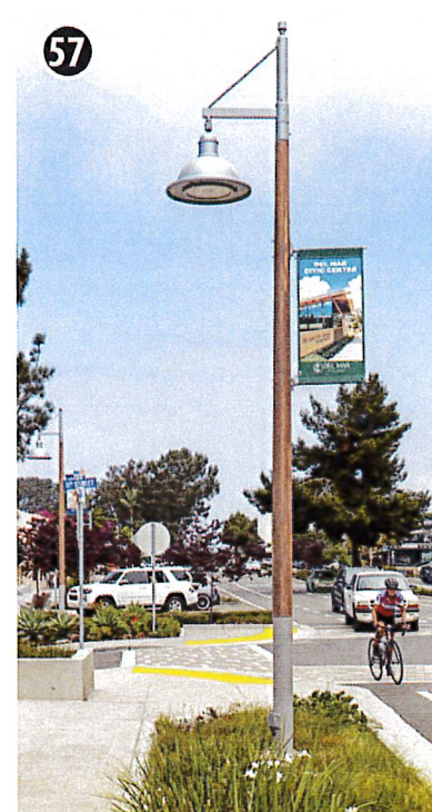
PEDESTRIAN / ROADWAY LIGHTING W/ WOOD POLE
